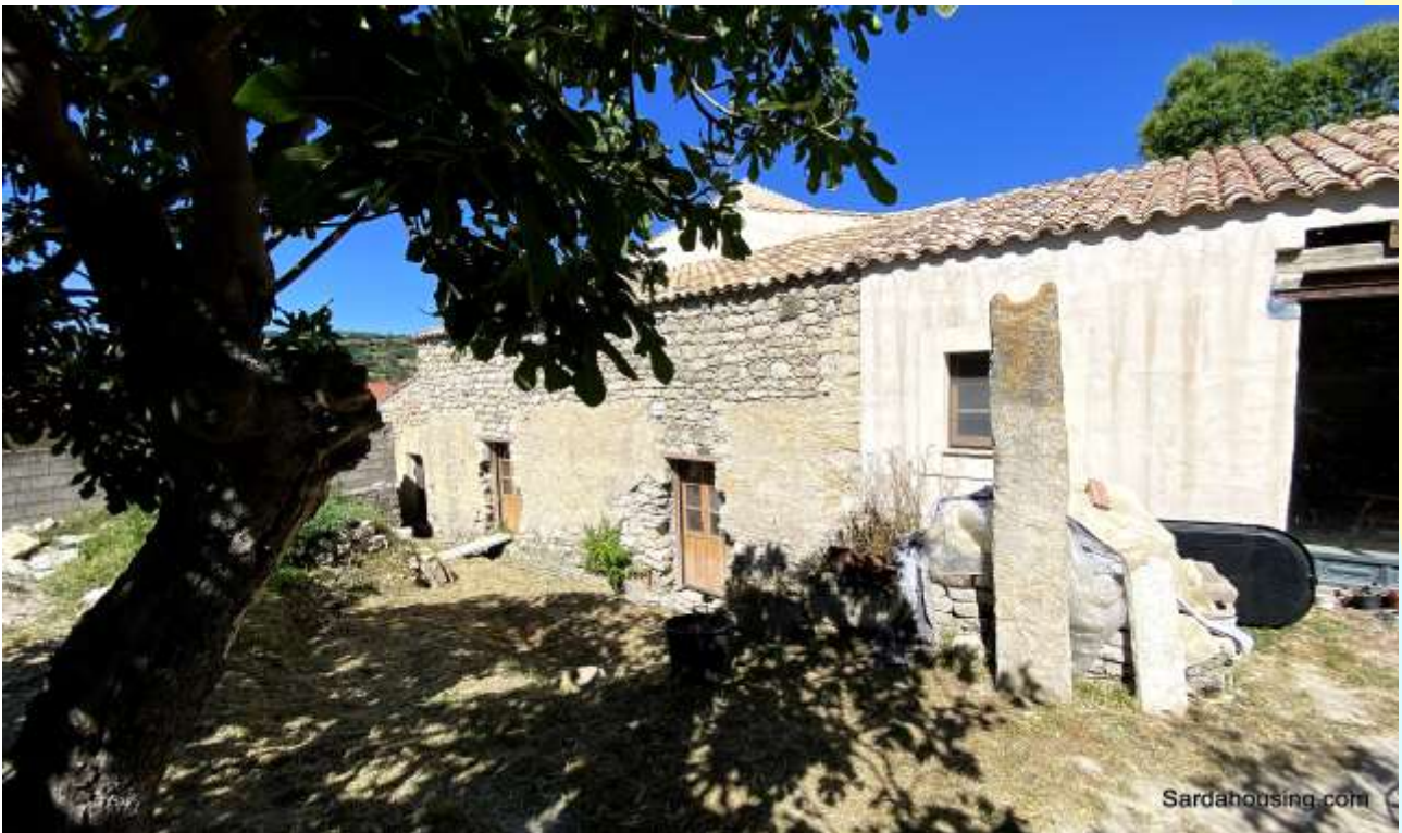
14 - Gesturi – Villa Regina Elena: garden and renovation works
