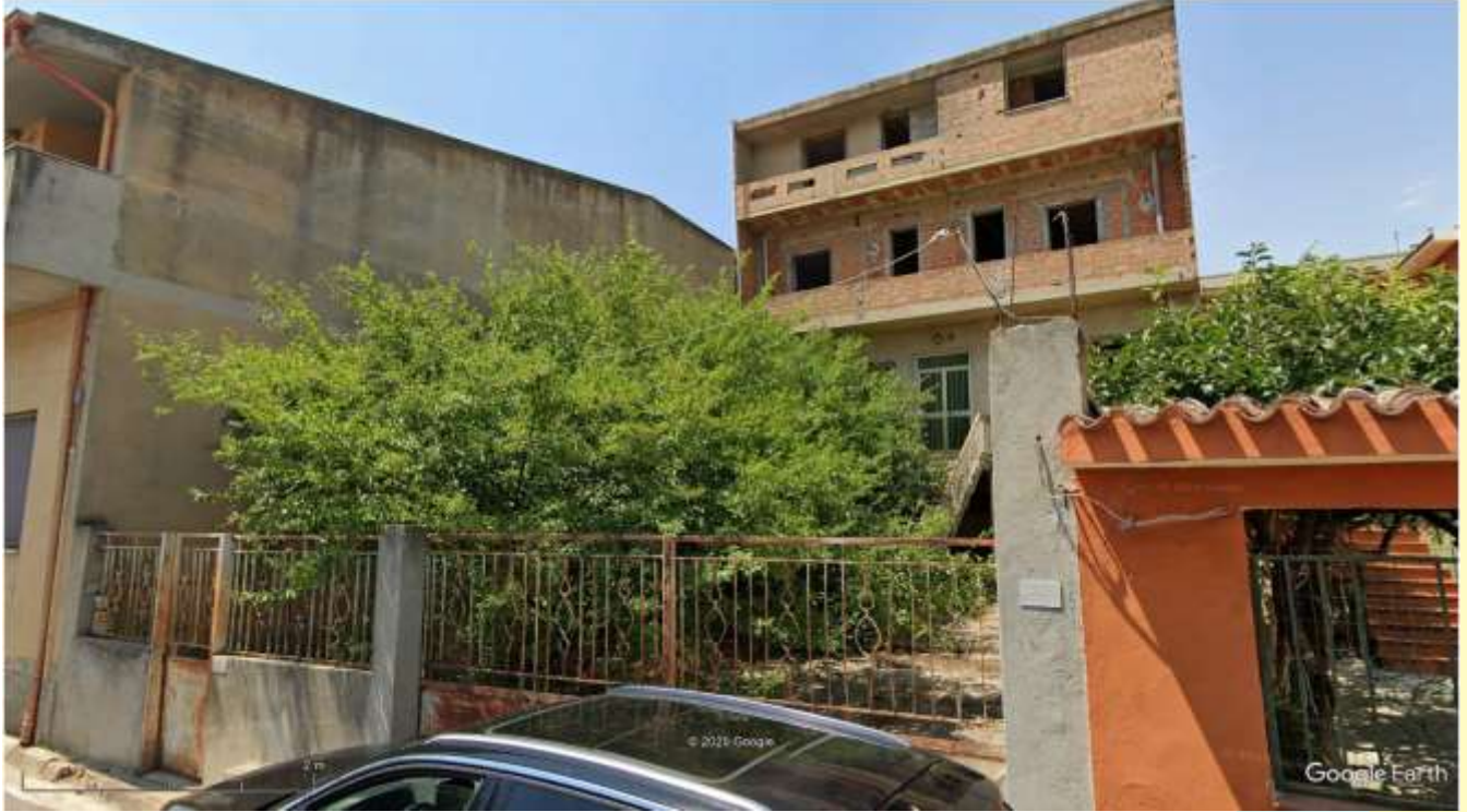
1 – Soleminis – Cagliari – Apartment Lussu on the first and second floors
