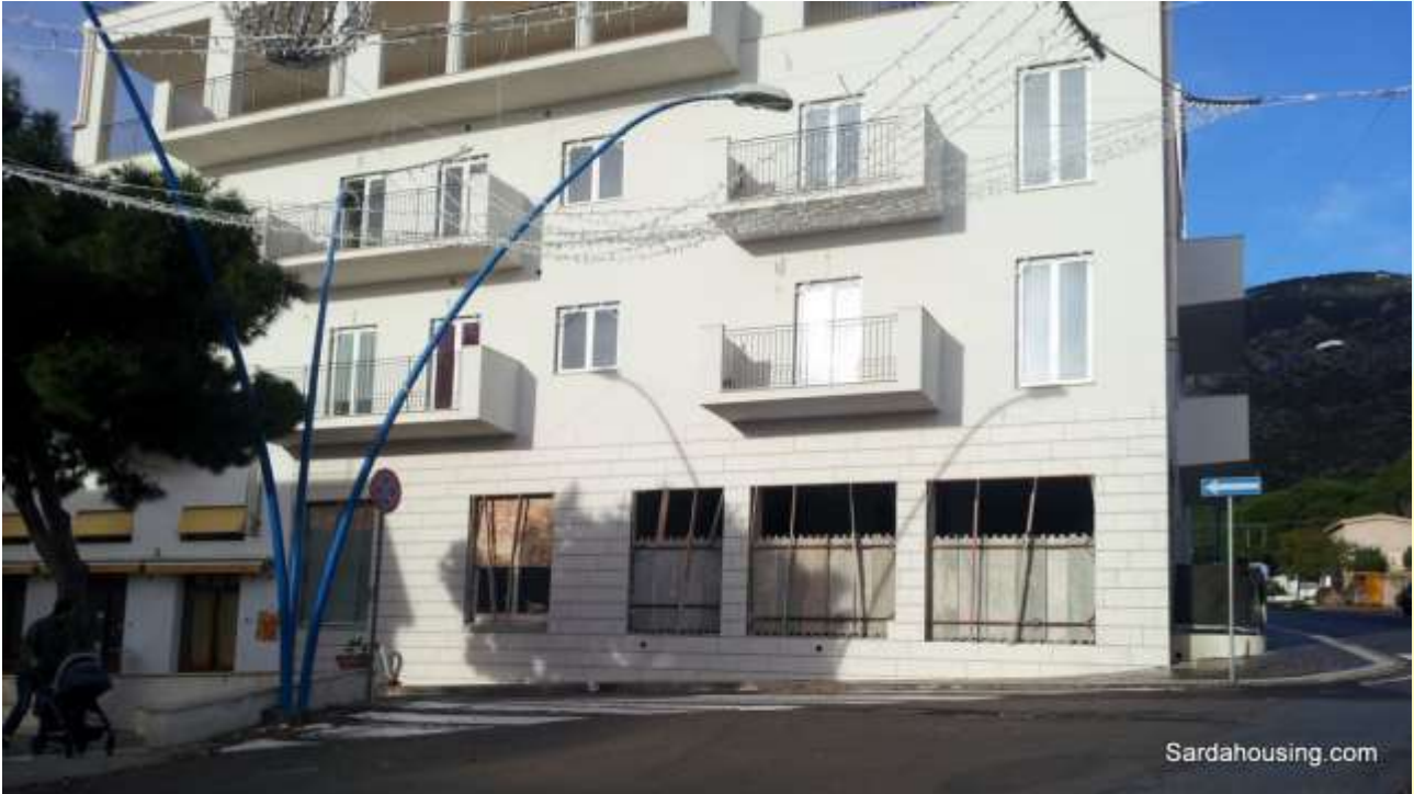
25 - - Cala Gonone – Dorgali – Penthouse Vasco – the renewed building
