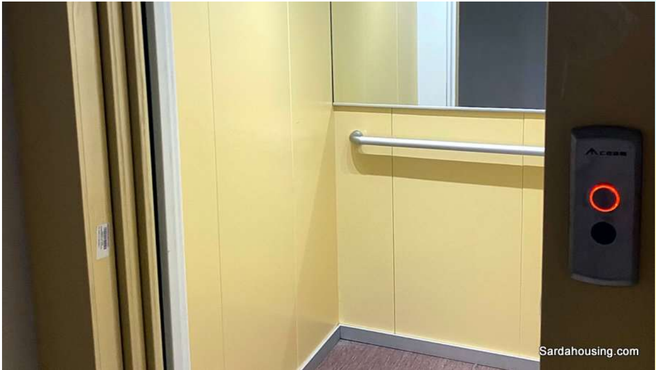
23 - Cala Gonone – Dorgali – Penthouse Vasco - lift
