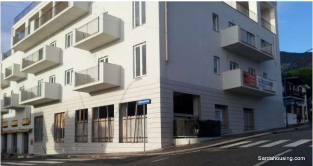
26 - - Cala Gonone – Dorgali – Penthouse Vasco – the renewed building
